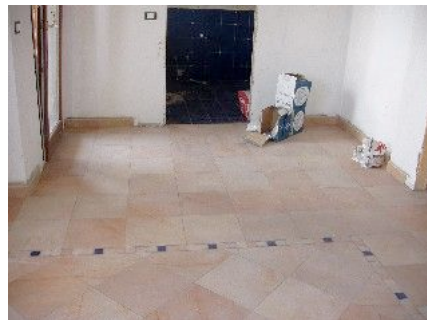
... and three days later - with the colour-schemed tiles and skirting tiles. Each suite and room has its own colour scheme and flower or fruit theme.
