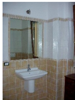
... and a completed shower room for one of the guest rooms (slightly smaller than the suites)
